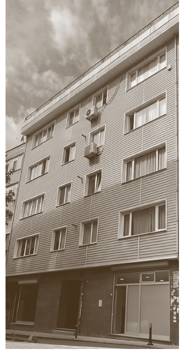
The house at number 2 on Kuyulubağ Street (today number 2-4, Akay Apartment). (Photo: Can Candan)
